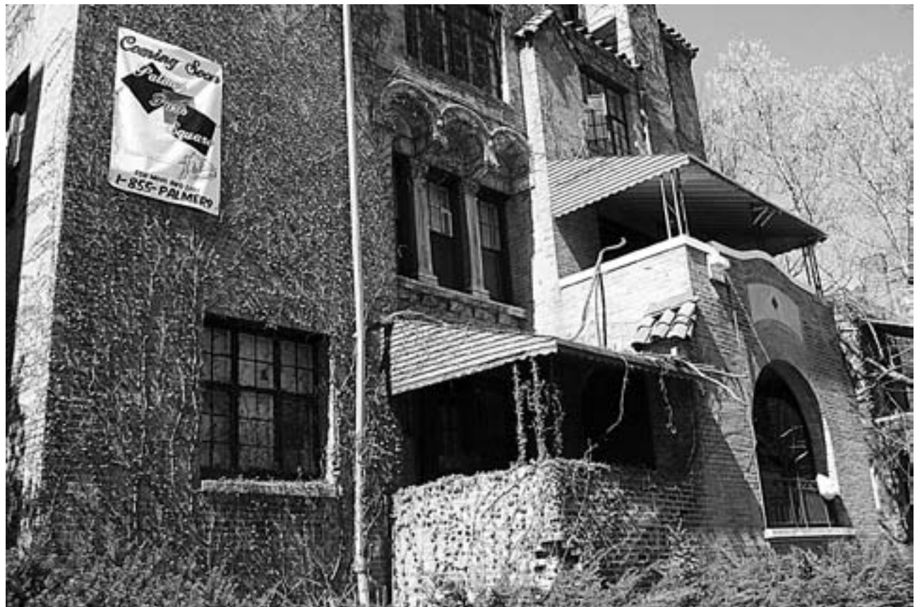
One of the six buildings that comprise the Palmer Park Square project currently under redevelopment by Shelborne Development. Photo: Jason A. Michael
