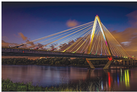
Bond Bridge in Kansas City
