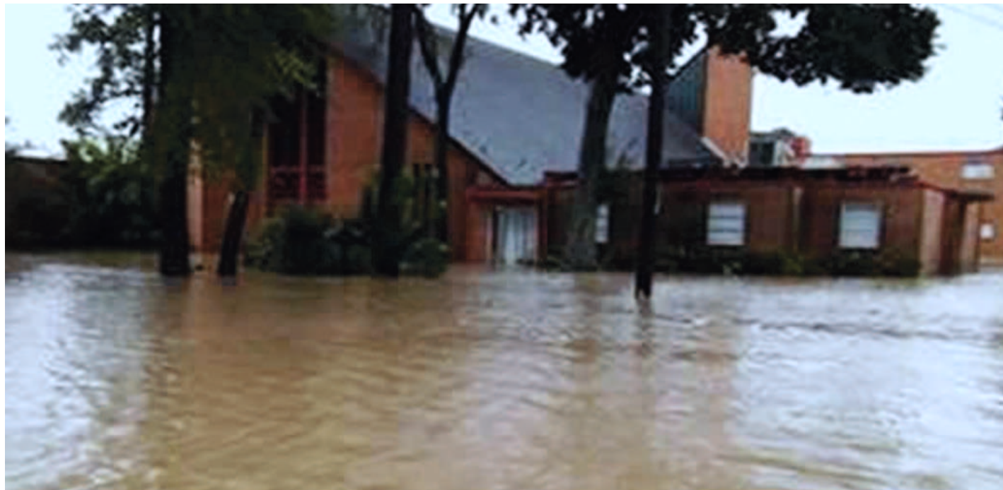
Floodwaters flood Resurrection Metropolitan Community Church in Houston on Aug. 27, 2017. What was once Hurricane Harvey has inundated large swaths of the city and southeast Texas since it made landfall on the state's Gulf Coast. Photo courtesy of Resurrection Metropolitan Community Church
